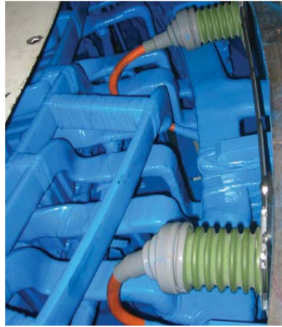
Couplers installed on a hydro generator stator
